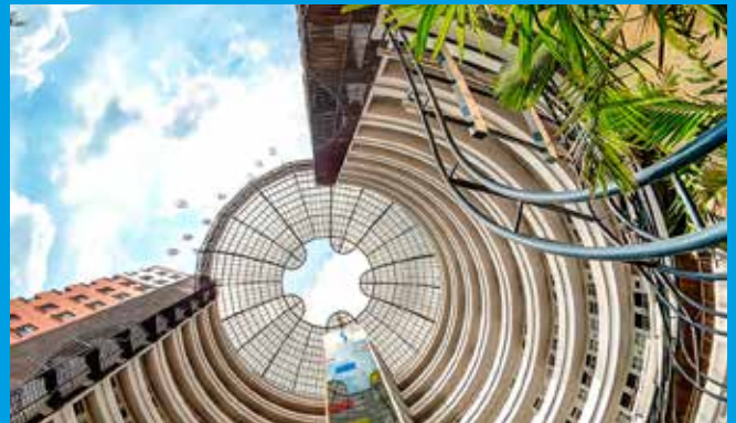
CENTRO COMERCIAL CHIPICHAPE, COLOMBIA
